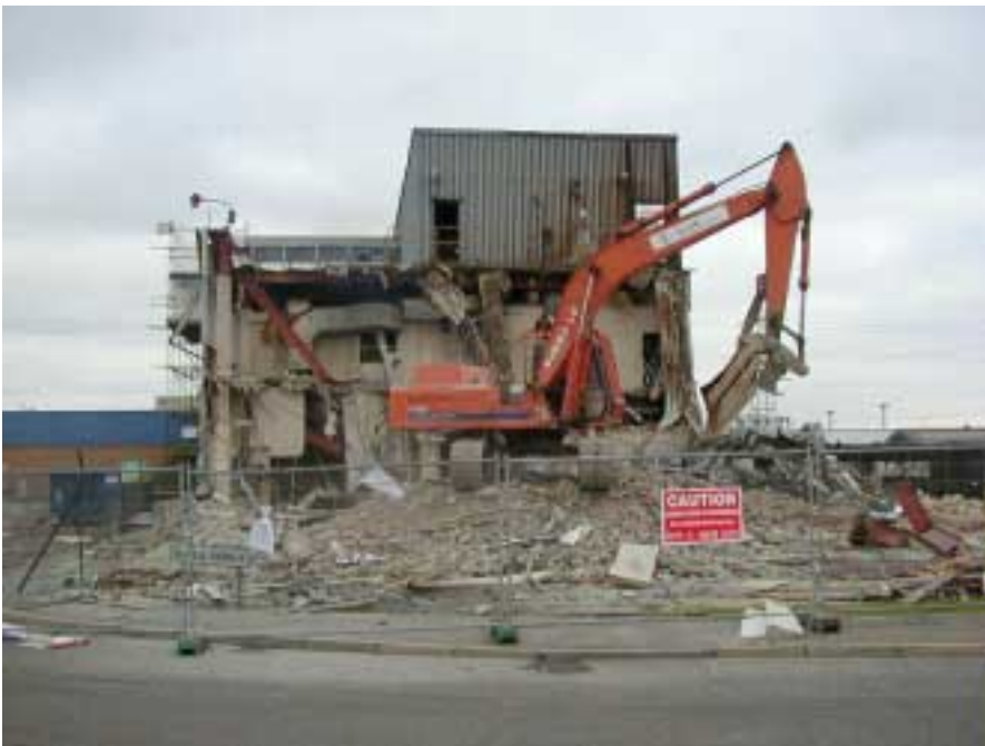
Demolition of disused office building at the former Ford, Dagenham site
